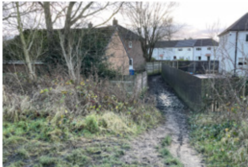
Impassable and hidden entrances
