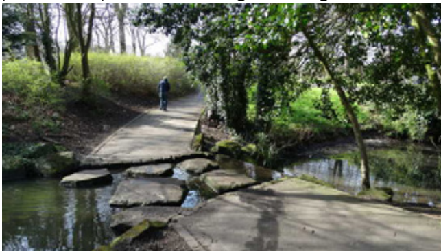
Footpaths retained open throughout the year by removing fallen branches, adding drainage, reprofiling, relocating, installing stepping stones
