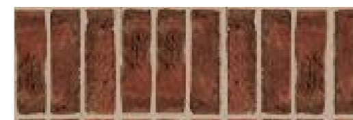
Soldier Bond Brickwork
