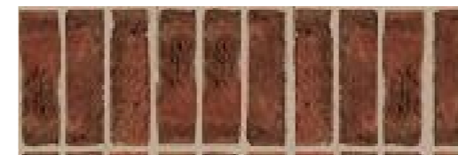
Soldier Bond Brickwork
